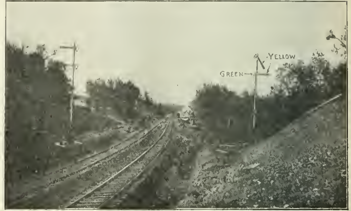
FIG. 9. RIGHT-HAND TRACK, FIRST BLOCK IN ADVANCE CLEAR, SECOND OCCUPIED—PROCEED CAUTIOUSLY.
